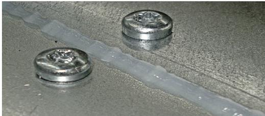
Figure 5-3 Applying silicone
