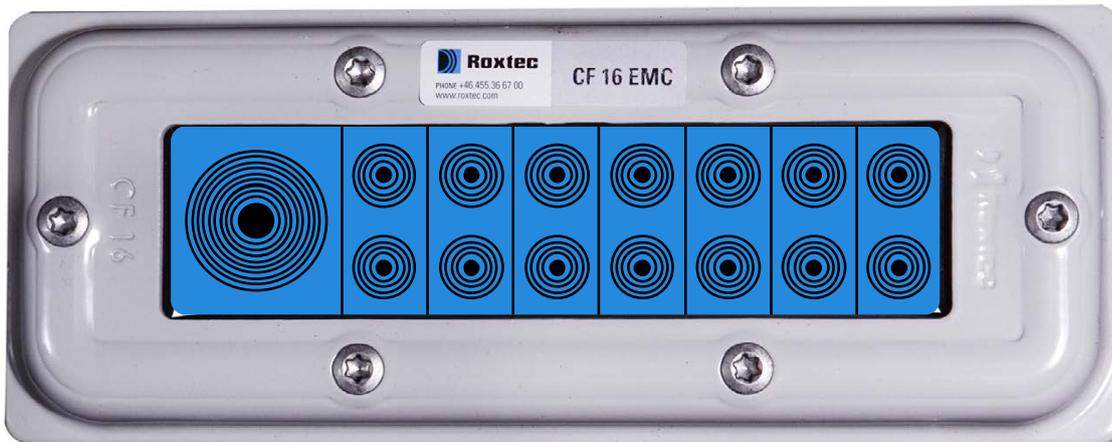
Figure 6-11 Cable entry with sealing modules – type 1
