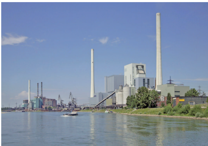
GKM power plant, Germany
