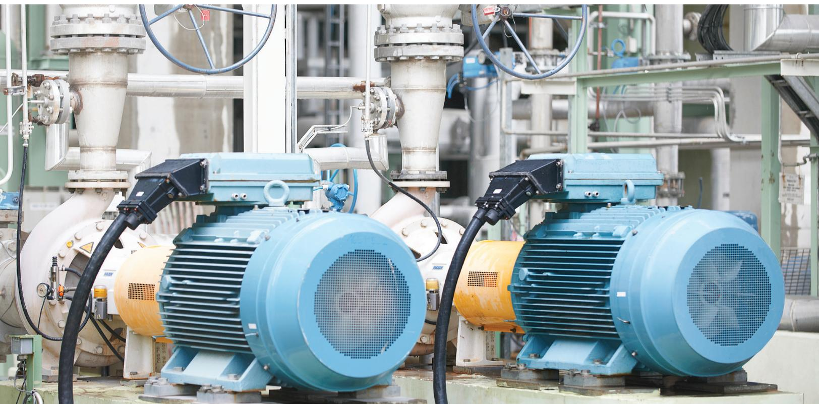
Electric motors consume about 65% of all electricity used throughout industry. Yet, less than 10% of those motors are fitted with a variable speed drive.
